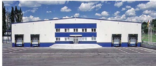
ZF Hungária Kft.: the heat-treatment facility in Eger
